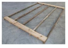
Step 2: Lay out remaining floor boards. Measure diagonals to ensure measurements are equal (i.e. floor is square). Rip down last floor board to suit gap, and nail off floor with 50mm flooring nails (10 nails per board).
