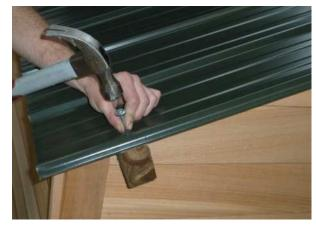
Step 17: Lay out remaining full roof sheets. Rivet these sheets together, 2 rivets per join, to make 1 large roof panel as shown in photo. Tack remaining top corner and bottom corner ensuring edge of sheet is flush with end of purlins and height is correct.
